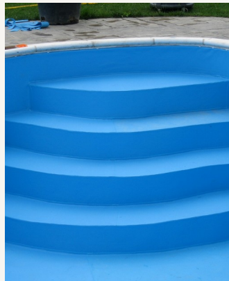
Stairs and finishes.
