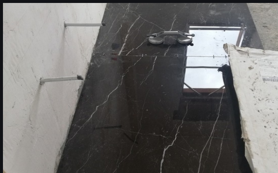
Latina • before refurbishment.
