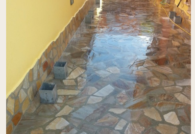
External paving • after.
