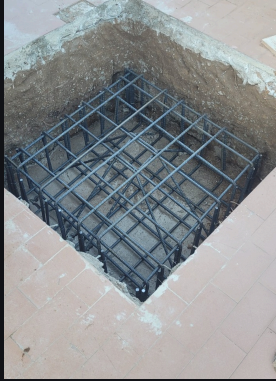
1 · Excavation and preparation.
