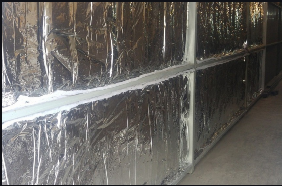
Wall framework and insulation.
