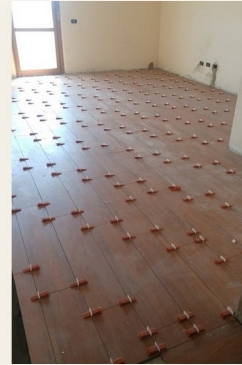
Floor installation • work phase.
