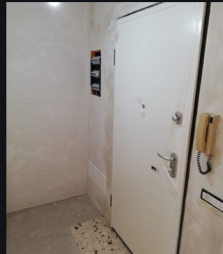
Entrance door · replacement and finishing.
