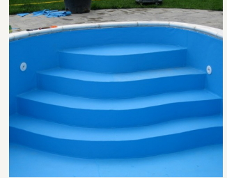
Completed stair detail.
