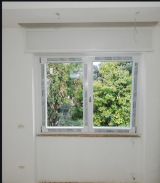
Window/door system + drywall · integrated works.
