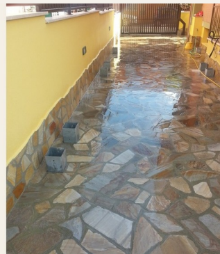
External paving • after.
