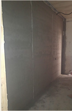
Preparation of surfaces and substrates.
