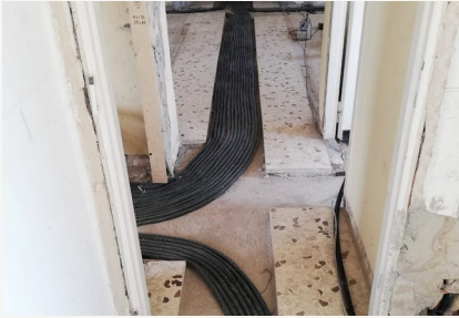
Distribution and installation of circuits.
